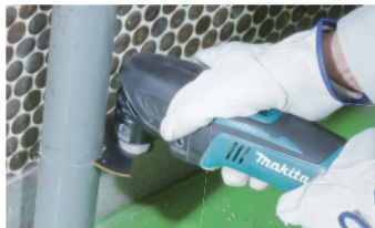
Routing joints on wall tiles
