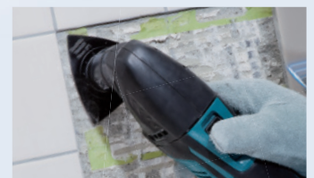
Removing mortar, tile adhesive
