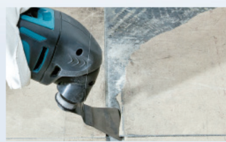
Scraping floor tiles
