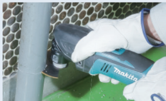
Cutting PVC, FRP pipes
