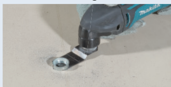
Metal flush cutting
