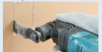
Cutting plasterboards
